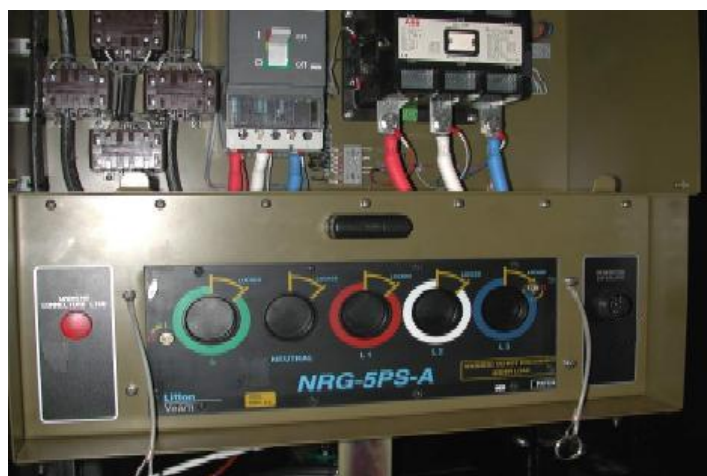
Figure 38C4-6:180 kVA/50Hz GPU Rear Power Panel
