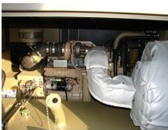
Figure 38B2-7: 120 KVA Pallet Mounted GPU's Engine Exhaust
