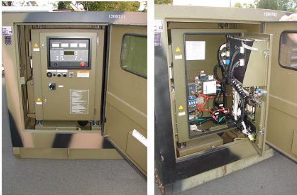
Figure 38B2-10: 120 KVA GPU's Control Panel and Rear Panel Electronics
