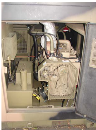
Figure 38B3-7: 60 KVA Pallet Mounted GPU's Engine Exhaust
