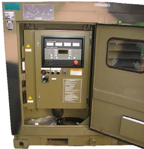
Figure 38B3-9: 60 KVA Pallet Mounted GPU's Control Panel
