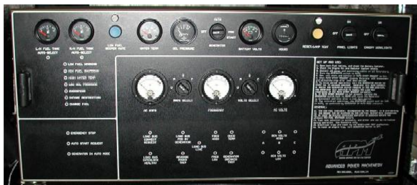
Figure 38C4-5:180 kVA/50Hz GPU Control Cabinet
