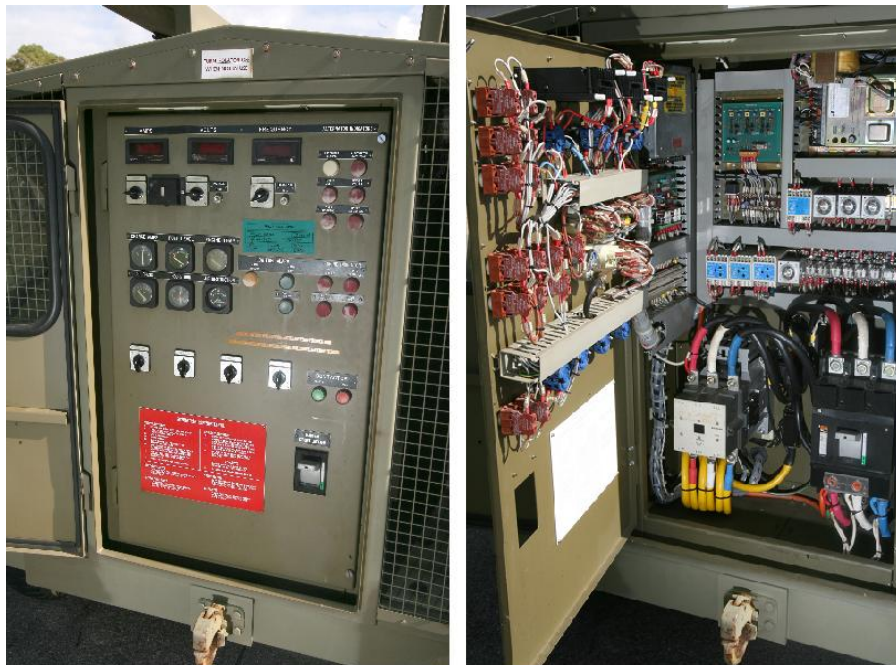
Figure 38A3-5: Modra 90 kVA GPU's Control Panel - External (Left) and Electronics (Right)
