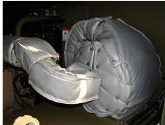
Figure 38B2-7: 120 KVA Pallet Mounted GPU's Engine Exhaust
